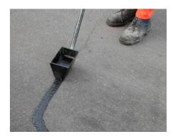
Jointgrip OB is an anti-skid overbanding joint sealant. It is a proprietary formulation of blended paving grade bitumen incorporating special polymers and abrasive aggregates to provide a compound of toughness, flexibility, adhesiveness and resistance to flow.
