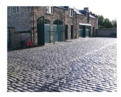
Sett Grout is a hot applied bituminous compound which secures all types of setts/cobbles. Sett Grout has been developed in order to solve the pouring and setting problems encountered with some filled bitumen grouting materials. Adhesion, flow and pouring properties have been improved whilst still retaining recommended softening point and penetration characteristics.
