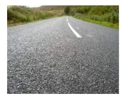
**Secure Chip** is a spray applied emulsion binder for application to recently completed surface dressings.
