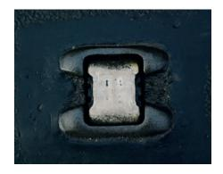
**Stud Grout** is a hot applied bituminous compound which secures reflective road studs.
