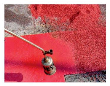
Antiskid Sheets are skid resistant thermoplastic sheets available in a variety of colours which are ideal for application on bus and cycle lanes as well as other high stress areas. Antiskid Sheets are easy to use, can be cut to size and are instantly trafficked once cooled. Antiskid Sheets are non-toxic, contain no lead or chromate pigments and are skid resistant to >55 SRV.
