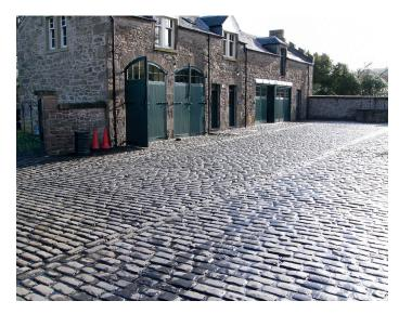
**Sett Grout** is a hot applied bituminous compound which secures all types of setts/cobbles. **Sett Grout** has been developed in order to solve the pouring and setting problems encountered with some filled bitumen grouting materials. Adhesion, flow and pouring properties have been improved whilst still retaining recommended softening point and penetration characteristics.
