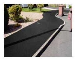
Cationic Slurry Seal Emulsion (CSS) is a key constituent of slurry seal for hand or machine application. Ideal for rejuvenating cracked, spalled and worn surfaces.
