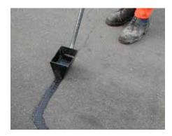
Jointgrip OB is an anti-skid overbanding joint sealant. It is a proprietary formulation of blended paving grade bitumen incorporating special polymers and abrasive aggregates to provide a compound of toughness, flexibility, adhesiveness and resistance to flow.
