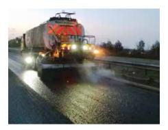
**Colbond Multi** is a polymer modified cationic bitumen emulsion designed to be applied both as a bond coat and vertical joint paint. **Colbond Multi** forms a uniform film of polymer modified bitumen on both horizontal and vertical faces forming a strong adhesive bond between bituminous overlay and the existing surface.
